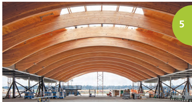
The new roof for the Portland International Airport, built using mass timber from Tribal and family-owned Pacific Northwest forests managing their lands to restore forest health. Photo credit: Stephen A. Miller, Courtesy of ZGF
